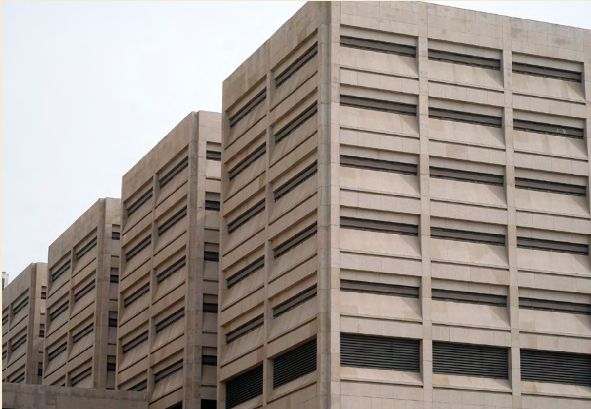
In a recording of a 911 call in December 2025, a Cuyahoga County jail employee asks for the address of the facility. GUS CHAN FOR THE MARSHALL PROJECT
