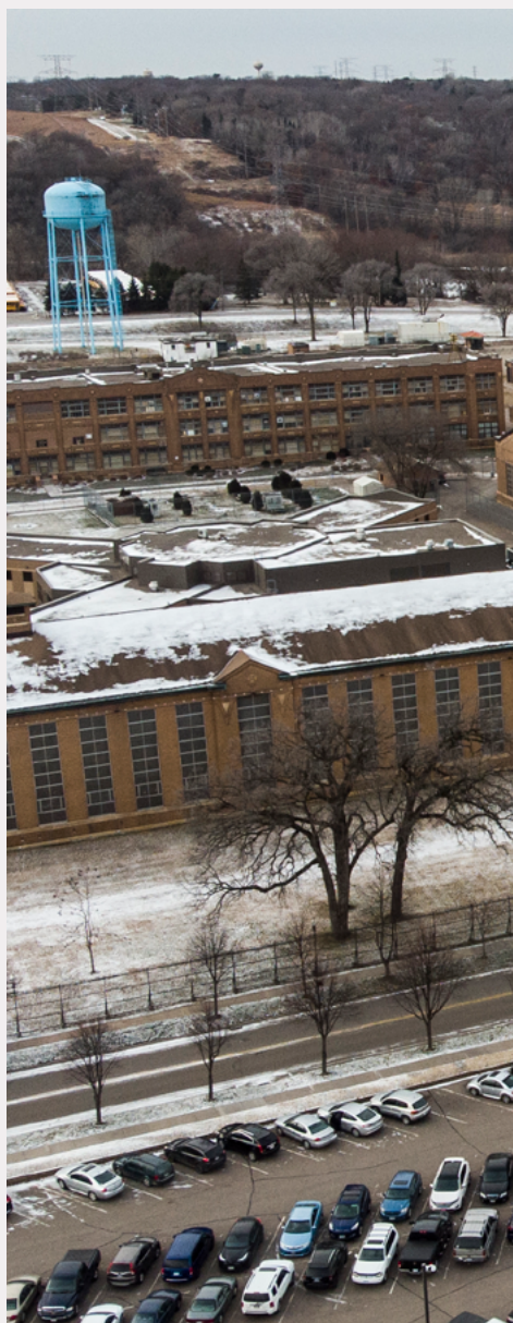
Minnesota Correctional Facility - Stillwater prison in Bayport, Minnesota, in 2020.
